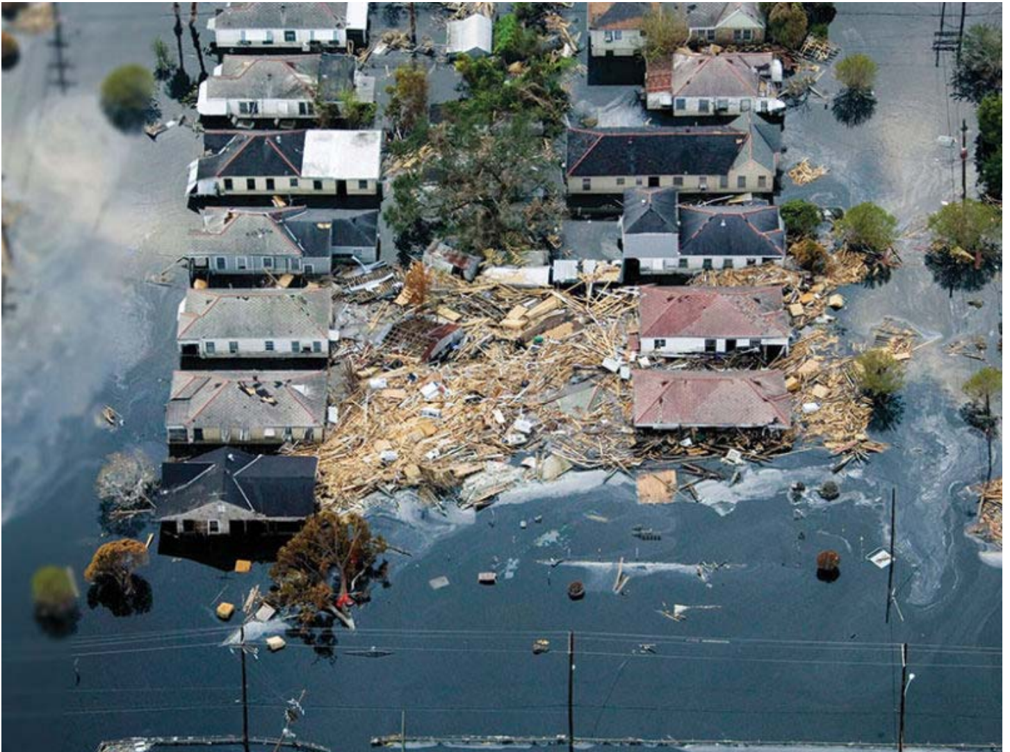
New Orleans, La., houses surrounded by debris and floodwater from Hurricane Katrina in 2005. Credit: Jerry Grayson/Helifilms Australia PTY Ltd/Getty Images
